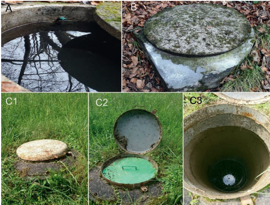
Fig. 1. Dug wells in the Nowy Sącz district (Southern Poland): A-C – different forms of dug wells (Photo. N. Nosal)
